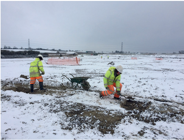
Plate 3.2 Site investigations on HRN3457 during snowy conditions
