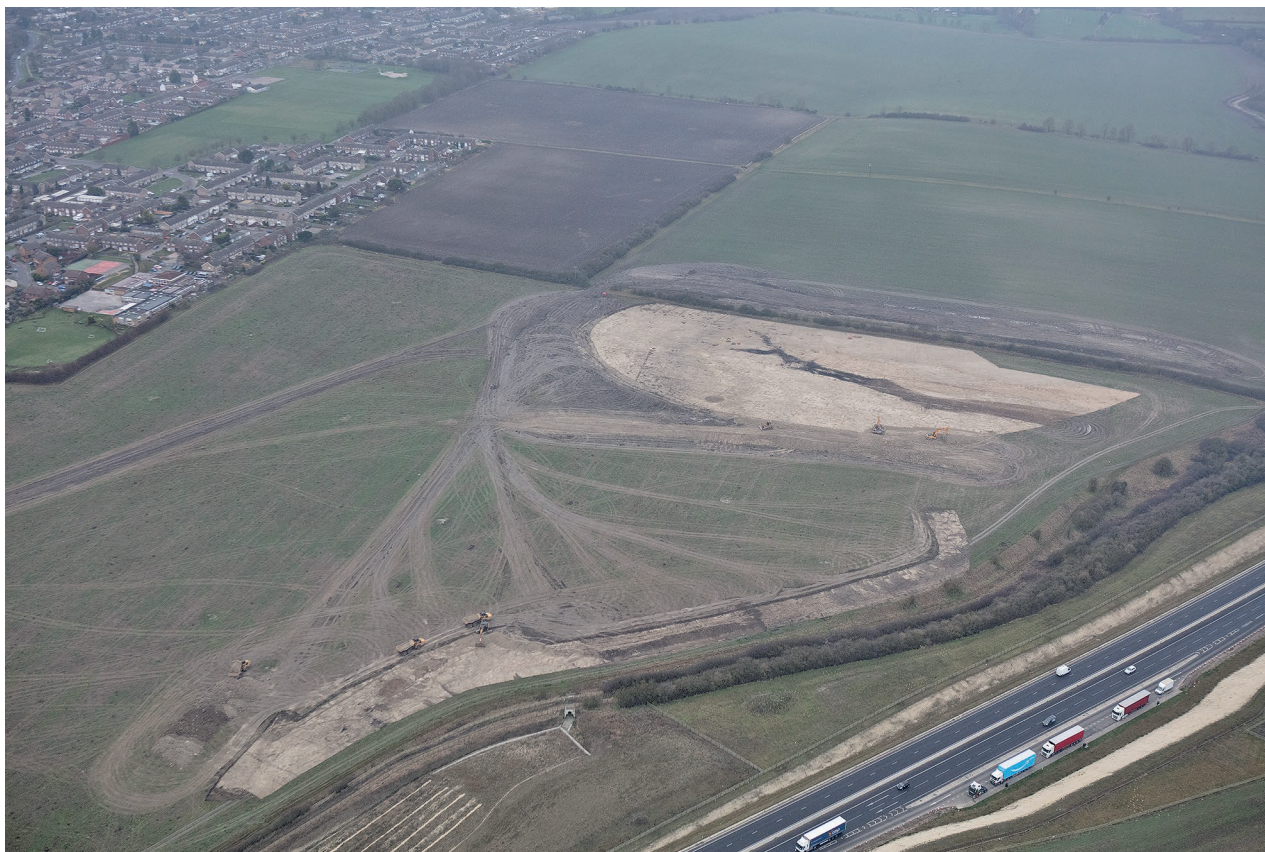
Plate 3.1 Aerial view looking west with HRN3457 in foreground (early in machining) and HRN3456 visible in centre, Houghton Regis on the left, and the Ouzel Brook and the A5–M1 Link Road on the right (January 2019)
