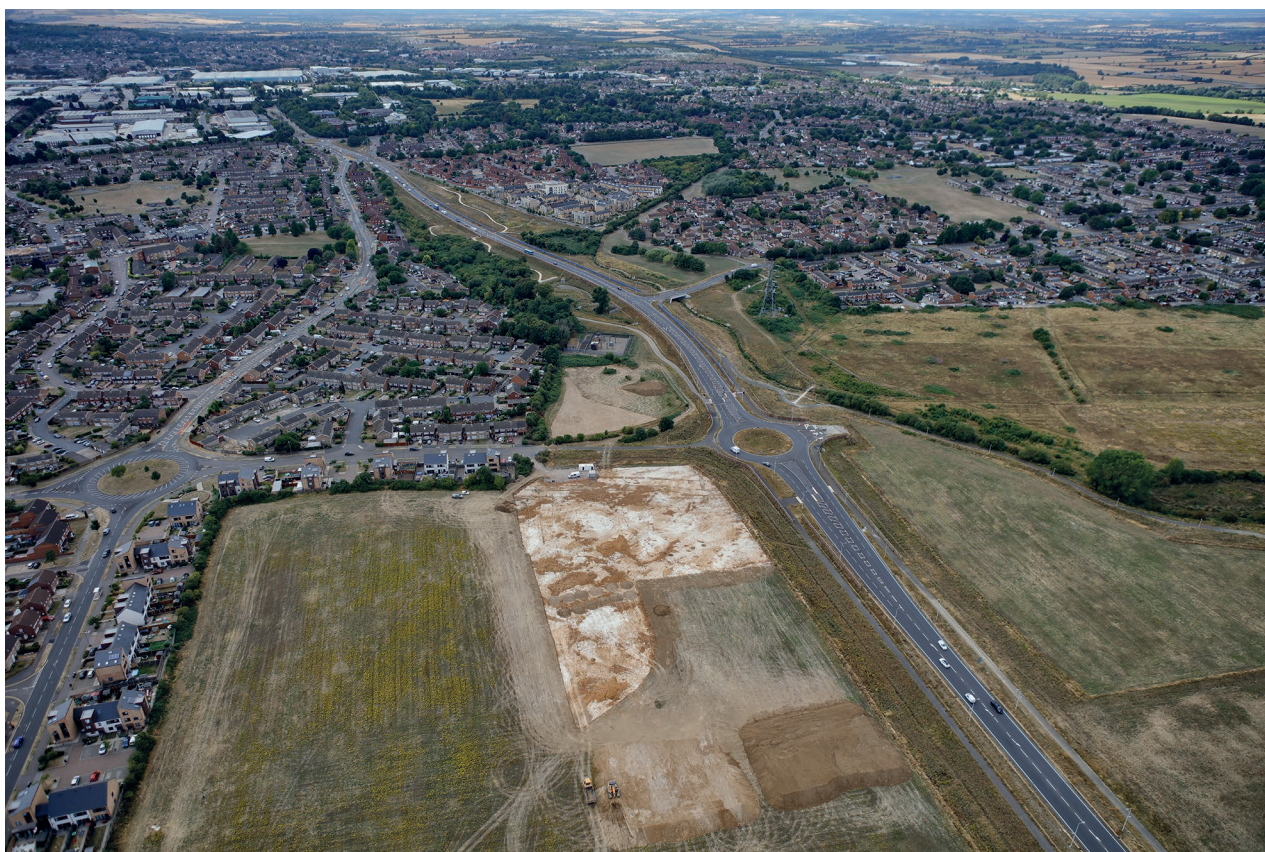
Plate 2.1 Aerial view looking west with HRN3205 visible in the foreground (west part backfilled) and Woodside Link on the right, beyond which is Houghton Regis and Dunstable (August 2018)
